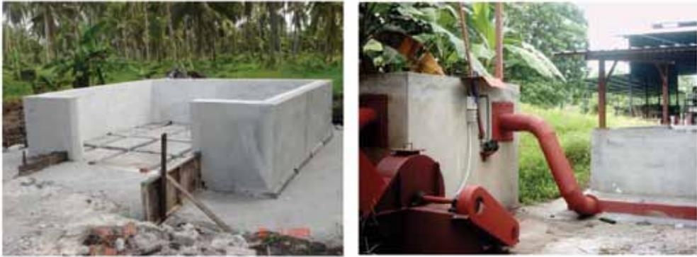
Figure 2. The building up of the hollow plinth brick carbonisation system.
