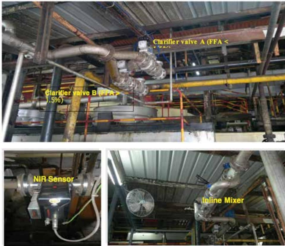
Figure 2. NIR Online System in the mill.
