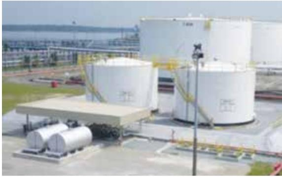
Figure 3. Installation of in-line blending facilities and two units of palm biodiesel storage tanks at a petroleum depot.
