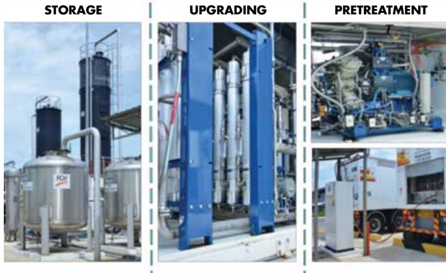
Figure 2. Main operation units of the bio-compressed natural gas (Bio-CNG) plant.
