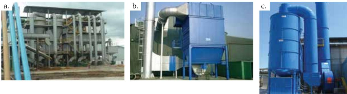
Figure 1. Types of particulate/dust control devices: (a) Cyclone separators, (b) Bag filters and (c) Wet scrubbers.
