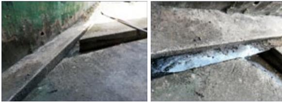
Figure 3. The premise compound was poorly maintained with oil clogging drain.
