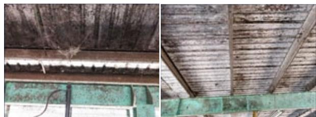
Figure 2. Roof and beams were rusty and dirty with cobwebs.
