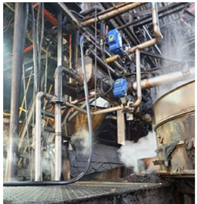
Figure 17. Dilution water control valves regulate accordingly to process requirement as computed in OBAMA panel.
