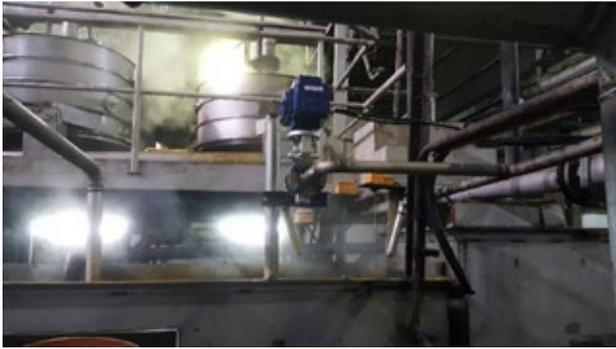
Figure 18. Recycle valve to manage constant over flow rate (OFR).
