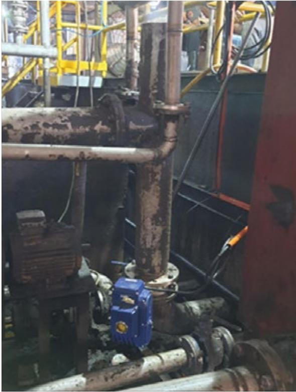
Figure 21. Level control valve at the SUF line responding to interface level transmitter.
