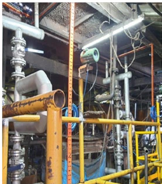
Figure 23. Vertically mounted flowmeters to promote self-draining effect measuring mass rate and fluid properties.
