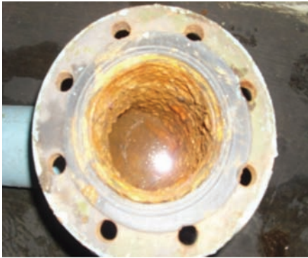
Figure 3. Inlet pipe to steam drum before installation of Merus ring technology.
