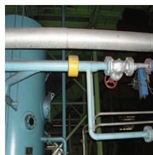
Figure 2. Installation of Merus ring technology at boiler feedwater pipe.
