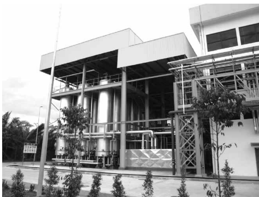
Figure 2. MPOB-Sime Darby winter-grade palm biodiesel plant.
