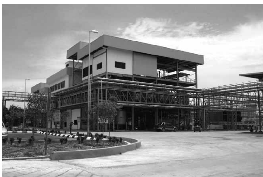
Figure 1. MPOB-Sime Darby normal-grade palm biodiesel plant.
