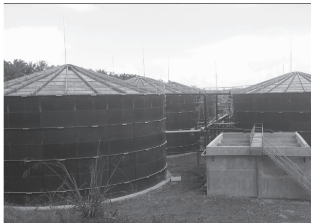
Figure 3. Biogas digester tank at Ladang Sabah Palm Oil Mill.
