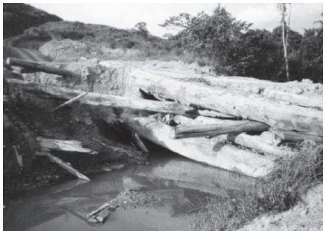
Figure 13. Collapsed crossing obstructing a stream channel.
