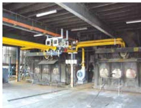
Figure 2. Biogas burners installed at palm oil mill biomass boilers.
