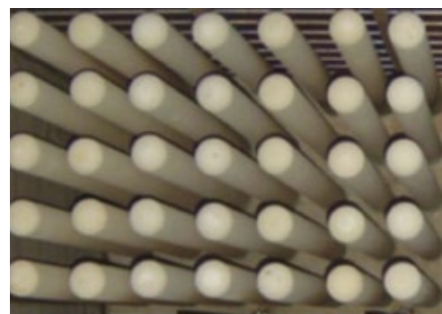
Figure 5. Hot gas installation.
